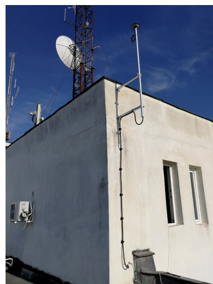
The antenna deployed at UPT.
